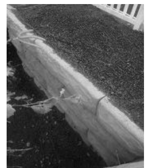
Top of retaining wall.
