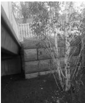
New retaining wall.
